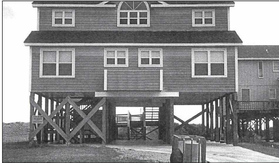
Figure 10-10. Diagonal bracing using dimensional lumber
