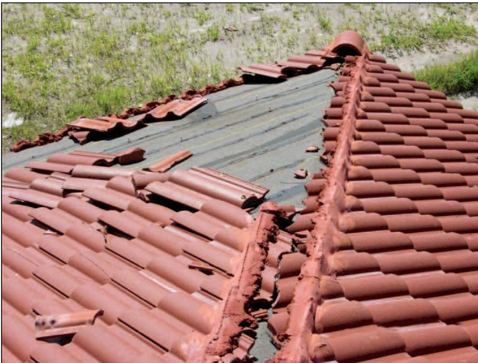
Figure 11-45. Blow-off of mechanically attached tiles. Estimated wind speed: 140 to 160 mph. Hurricane Charley (Florida, 2004)
