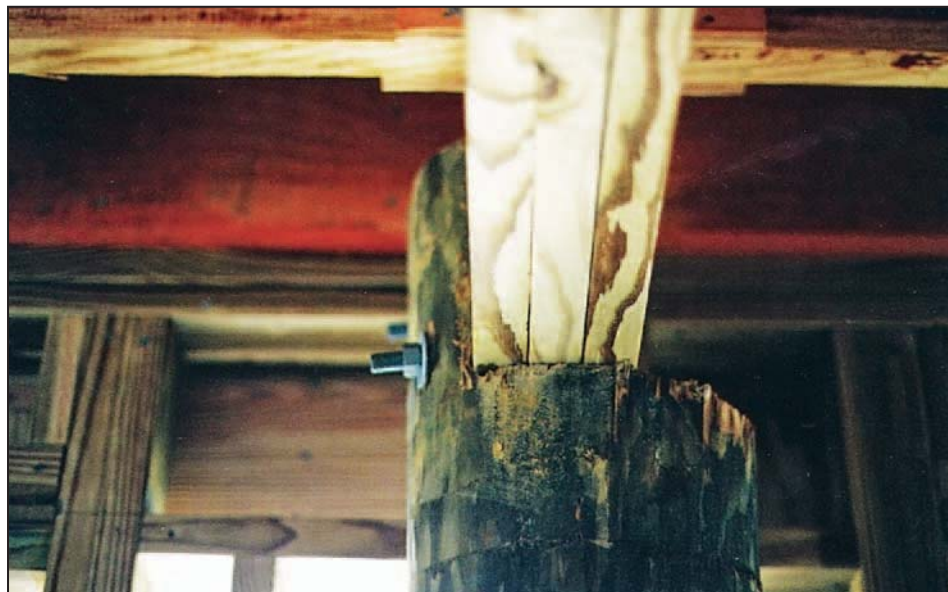
Figure 13-3. Improper overnotched wood pile
