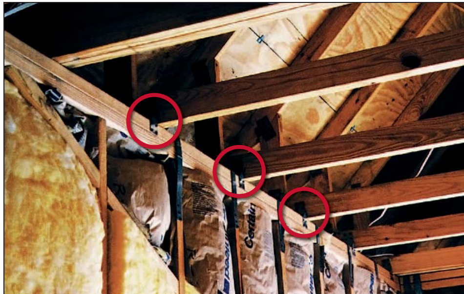
Figure 9-9. Connection of truss to wood-frame wall
