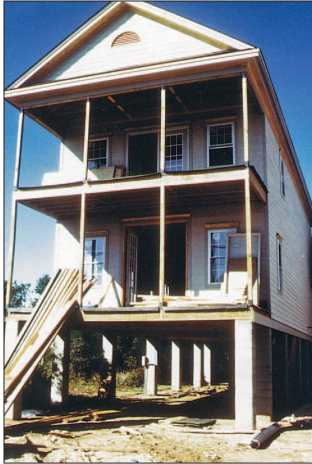
Figure 13-6. Open masonry foundation
