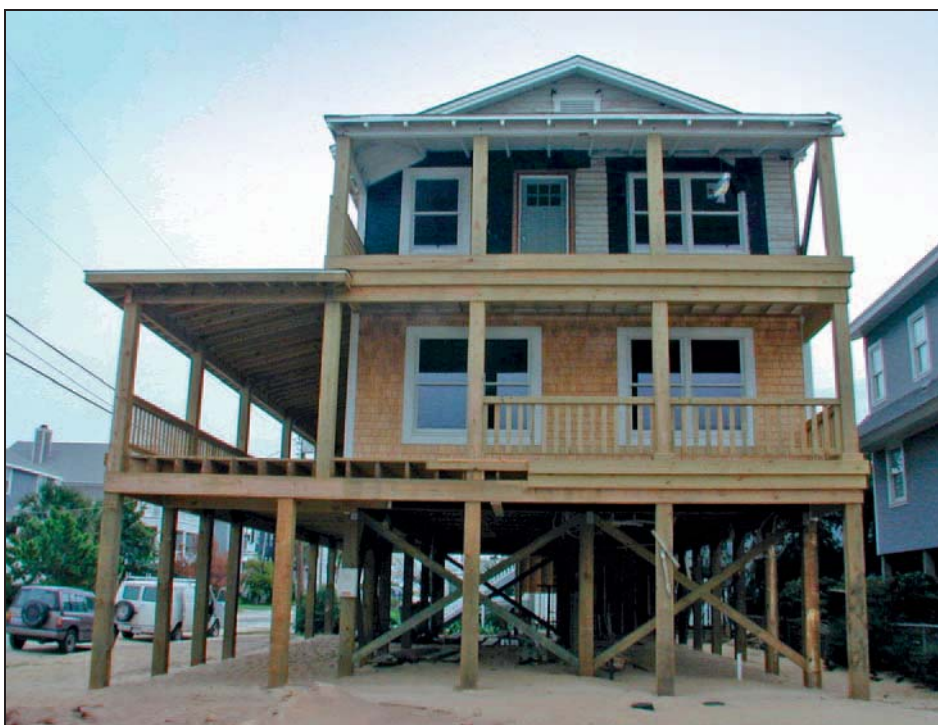
Figure 15-9. Home elevated on piles
