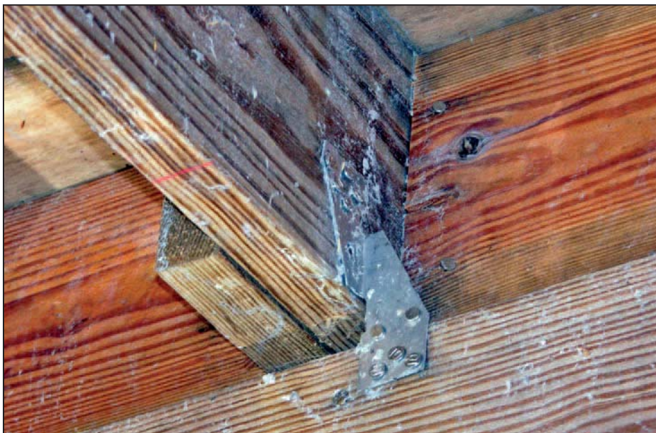
Figure 9-17. Metal joist-to-beam connector
