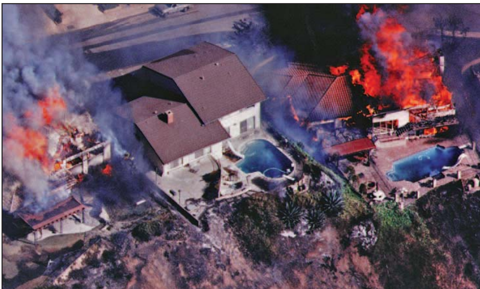
Figure 11-3. House that survived a wildfire due in part to fire-resistant walls and roof while surrounding houses were destroyed SOURCE: DECRA ROOFING SYSTEMS, USED WITH PERMISSION
