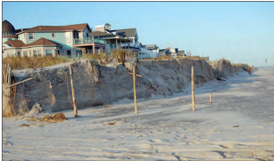
Figure 3-31. Dune erosion in Ocean City, NJ, caused by the remnants of Hurricane Ida (2009) and a previous nor'easter
