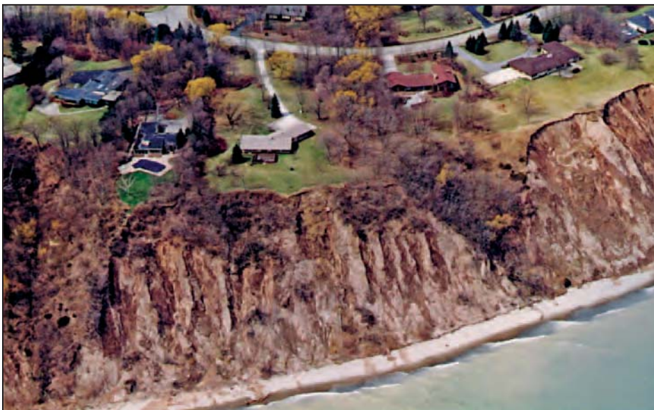
Figure 3-46. Long-term erosion of the bluff along the Lake Michigan shoreline in Ozaukee County, WI, increases the threat to residential buildings outside the floodplain (1996 photograph)
