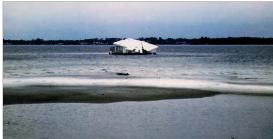
Figure 3-22. This house, located in an area of channeled flow near that shown in Figure 3-20, was undermined, washed into the bay behind the barrier island, and became a threat to navigation
