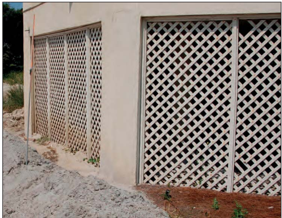
Figure 2-22. An enclosure formed by open lattice (Isle of Palms, SC)
