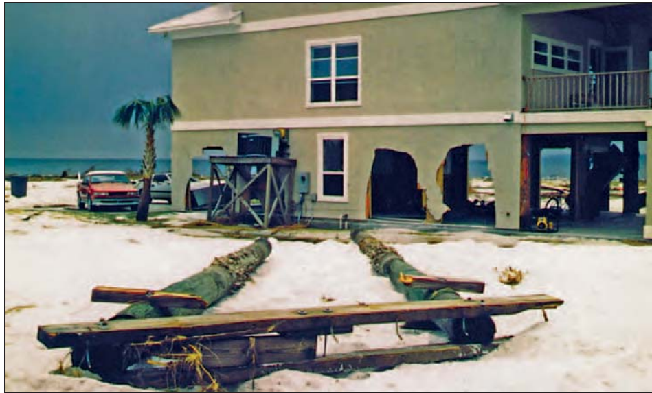
Figure 3-28. Pier pilings were carried over 2 miles by storm surge and waves before they came to rest against this elevated house in Pensacola Beach, FL (Hurricane Opal, 1995)
