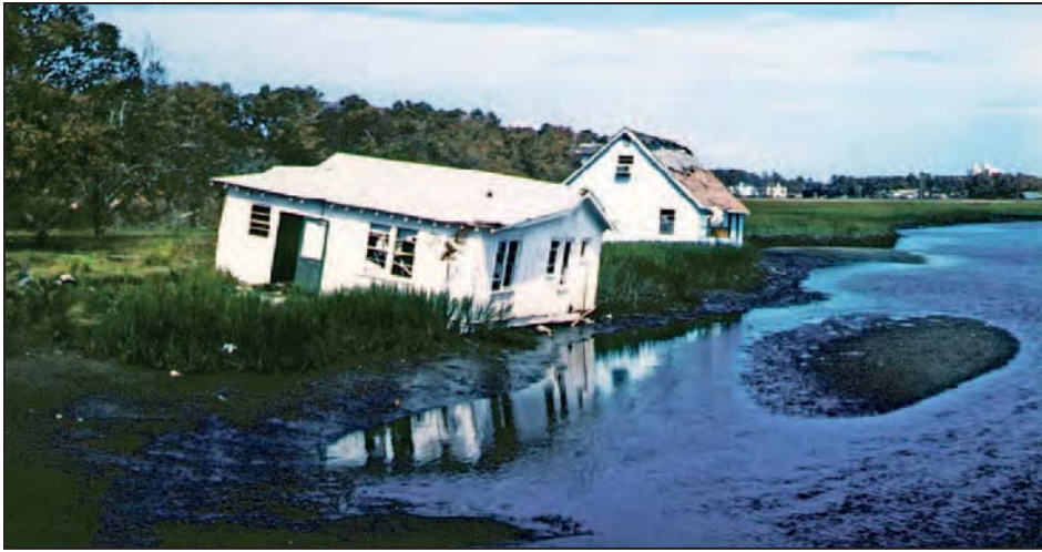
Figure 3-18. Intact houses floated off their foundations and carried inland during Hurricane Hugo in 1989 (Garden City, SC)
