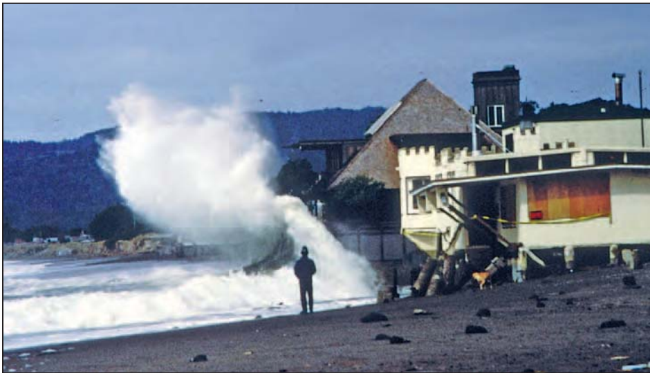
Figure 3-23. Storm waves breaking against a seawall in front of a coastal residence at Stinson Beach, CA SOURCE: LESLEY EWING, USED WITH PERMISSION
