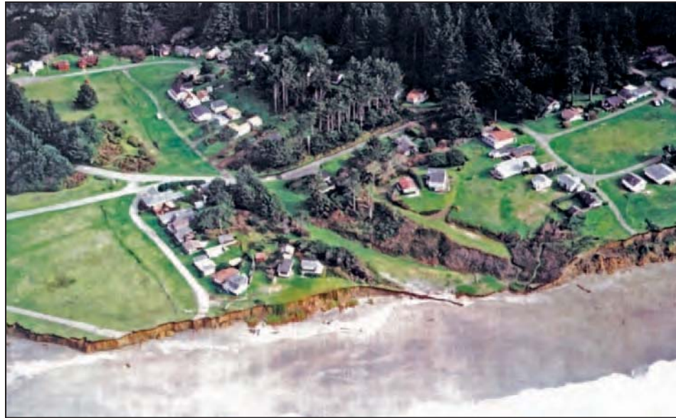
Figure 4-19. As buildings in this Humbolt County, CA, community are threatened by bluff erosion along the Pacific Ocean, they are moved to other sites on the jointly owned parcel
