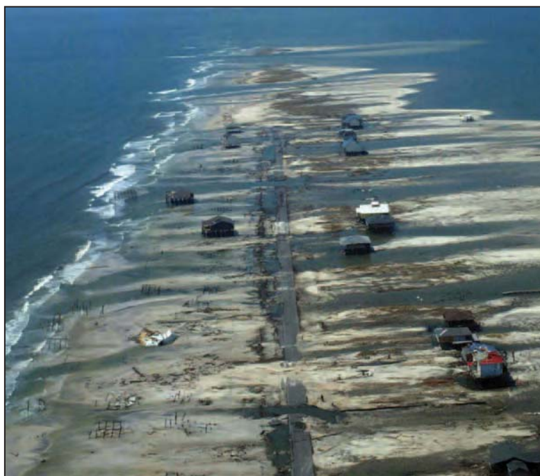
Figure 4-16. Narrow, low-lying areas and barrier islands (such as Dauphin Island, AL, shown in the photograph) are routinely subjected to coastal storm effects (Hurricane Katrina, 2005) SOURCE: USGS
