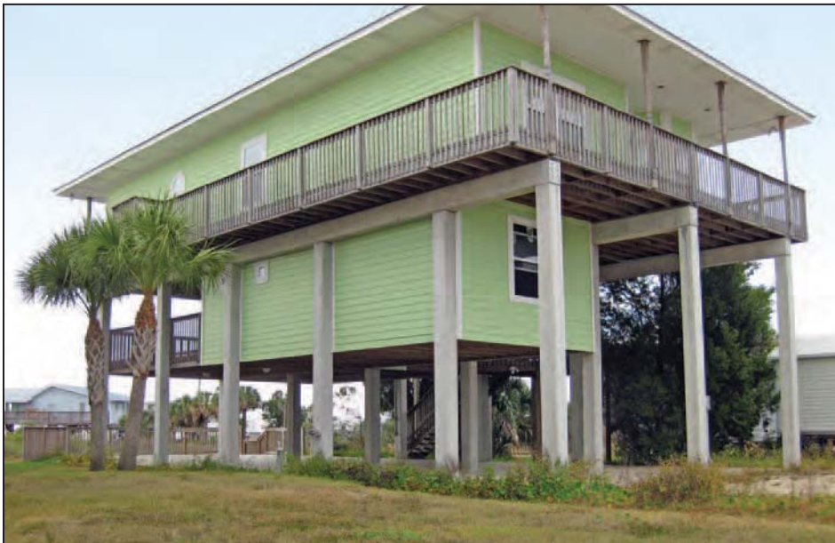
Figure 2-23. Above-grade enclosure (Perry, FL)
