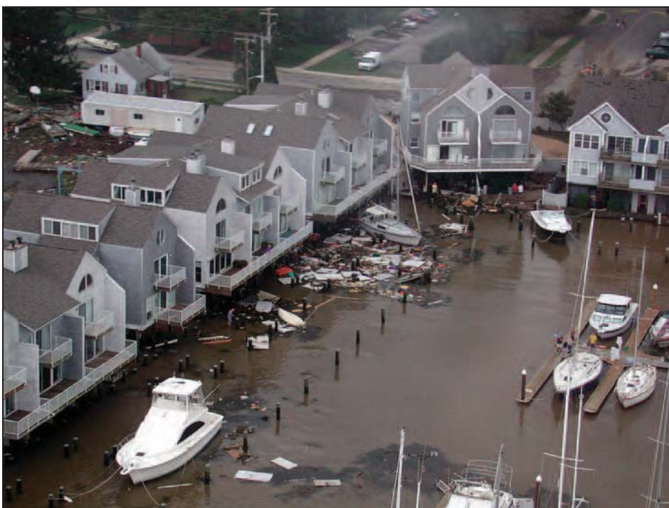
Figure 4-21. Condominiums built along the shoreline at the mouth of the Susquehanna River on the Chesapeake Bay were subjected to flood-borne debris after Hurricane Isabel (Havre de Grace, MD, 2003)
